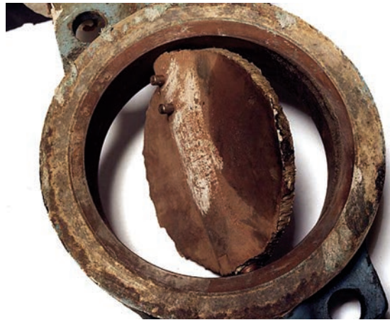
FIGURE 9. CAVITATION DAMAGE TO BUTTERFLY VALVE
